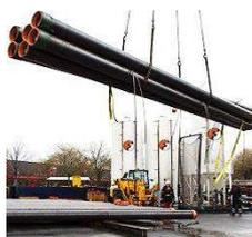
The Paris Basin is known for its geothermal energy recovery installations. The challenge in this area is the low fracture gradient of the formation. To allow economic hot water flow rates, large diameter strings which cover long intervals need to be cemented in place. A French operator turned to FES where a project required slurry densities of 1,20 SG. The HOZlite system designed, allowed the successful casing isolation to surface with a 1650 PSI compressive strength development.
